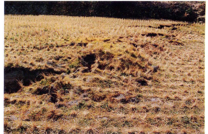
写真11. 地点⑯. 開口亀裂と地表変位 Photo. 11 Flexural deformation and extensional cracks at Loc ⑯
