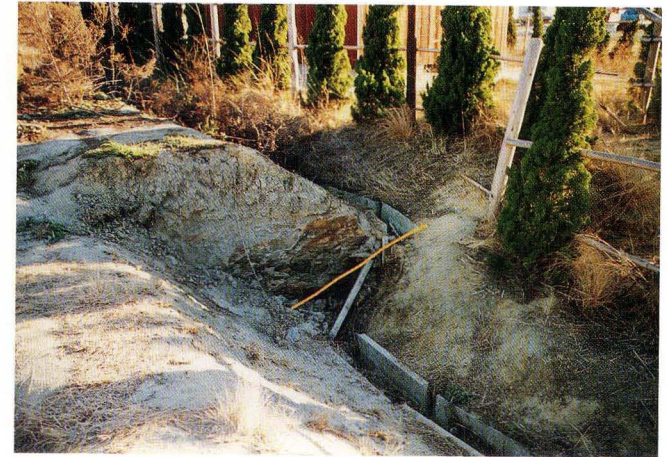
Photo. 51 Right lateral offset of waterway at Loc ⑦⑥
