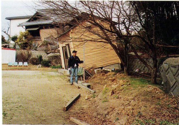
写真57. 地点⑧③. 丸太小屋直下を通過した断層 Photo. 57 Tilted loghouse passed by surface fault at Loc ⑧③
